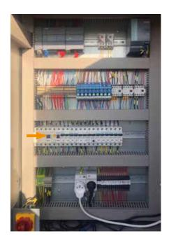
1 Check the redisual-current circuit-breaker with the TEST button (if works properly, the machine should be switched-off).
