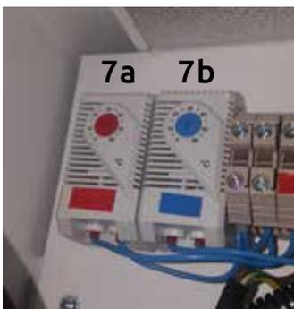
3 When the power is switched-on, proper operation of air heater and cooling fan should be controlled. For this purpose set the temperature of 7a thermostat above the ambient temperature, the heater should start to work. After 1 minute the heaters should be noticeably warm. Restore the old temperature setting. The same procedure needs to be done with thermostat 7b, although set the temperature below the ambient temperature. If the fans start to work, the old temperature setting can be restored.
