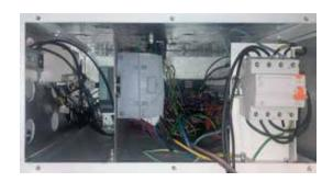
1 Check the redisual-current circuit-breaker with the TEST button (if works properly, the machine should be switched-off).
